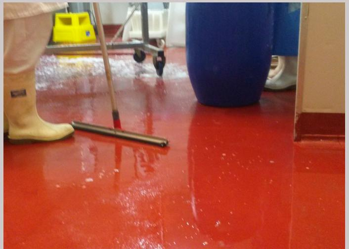
**Cleanability** - This comes from the combination of correctly installed floor slopes, an impermeable flooring material that is not overly hard to clean coupled with the right cleaning processes. Floor to wall junctions must be coved to ease cleaning.
