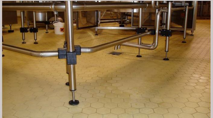
**Corrosion Resistance** - all foodstuffs are corrosive. The worst food areas are where hot fats are in frequent contact, and poultry fat is the most aggressive. All components of the flooring system must be designed to resist corrosion or the result will be impossible to clean floors firstly, thereafter unstable corroding floors not fit for purpose.
