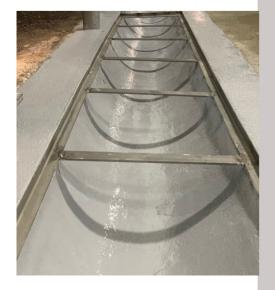
The drain & surrounding floor areas at this food production facility were heavily corroded and in need of urgent repair.
